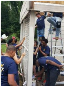
Stockbridge High School FFA members repainting a local house
